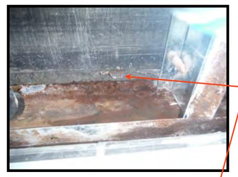
THE EXPOSED MUD DECK OF THE EDGE OF THE SHOWER FLOOR, THIS AREA SHOULD OF HAD A CLOSURE STRIP OR "L" METAL THE STOPS THE FLOW OF THE WATER AT THE PAN.
