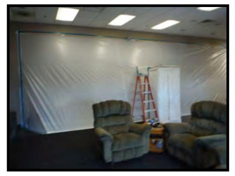
WCRC INSTALLED A POLY CONTAINMENT TO ALLOW FOR CONTROLS WHILE REMOVING THE AREAS DAMAGED FOR INSPECTION AS NEEDED.
