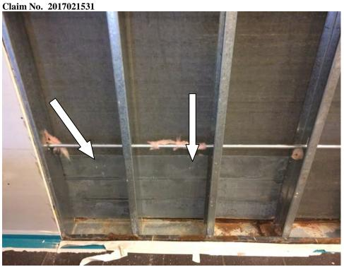
Above is the back of the wall in the area where the bench is installed. You can see the installed screws which punch through the metal in the areas noted by the arrows. There is no evidence of water coming through the wall through these openings that I can see.
