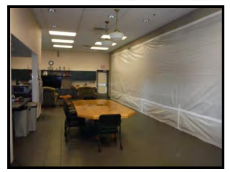
WITH THIS PHASE OF THE REPAIR COMPLETED AND TESTED WCRC REMOVED THE CONTAINMENT AND INSTALLED POLY OVER THE COMPLETE WALL.
