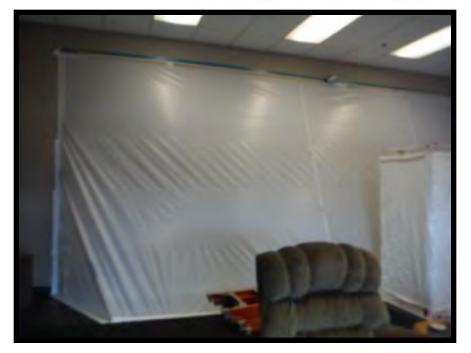
DUE TO CEILING HEIGHT WCRC INSTALLED CONTAINMENT TO WALL FOR THIS PHASE OF THE WORK.
