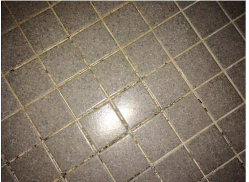
Above is a photo showing the condition of the bathroom tile, though to potentially be the second possible source of water. In this photo you can see the grout between the individual tiles is worn down and, in some areas, entirely gone. This is an exemplar photo, and does show one of the worst single areas, but grout maintenance is an issue over all of the installed tile.
