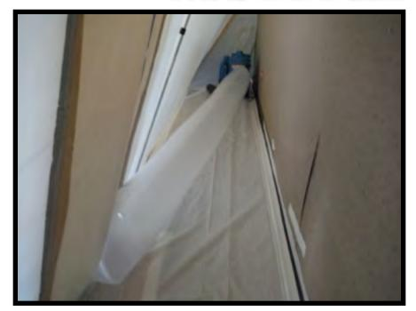
LAY FLAT DUCTING BEING INSTALLED, THE DUCTING WILL EXIST OUTSIDE OF THE CONTAINMENT AND BUILDING.
