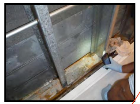
WITH THE WALL EXPOSED WCRC WATER TESTED THE SHOWER.
