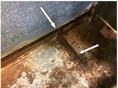
Above is a view of this area up close. There is an area of overlapping sheet metal here, and the water comes between these sheets into the pan formed by the sill. During the water test this area started to get moist, and then wet, over the course of 20 minutes.
