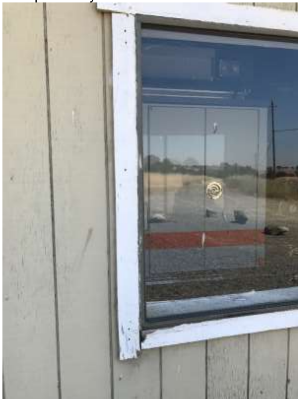
Example of Dry Rot On Exterior
