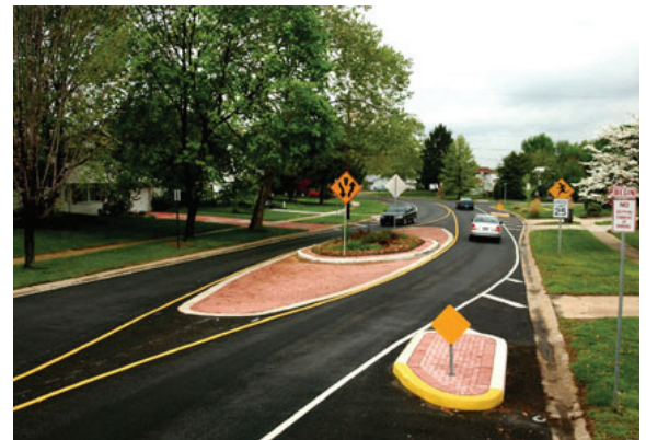
Examples of Effective Horizontal Deflection Traffic Calming Device: Medians
