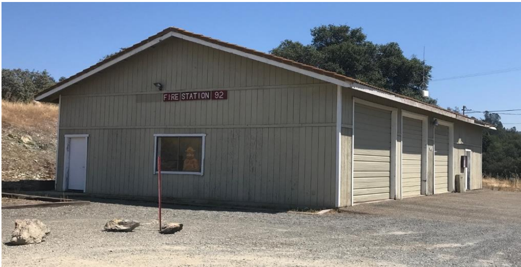
Station 92 – 7470 Ryan Ranch Road
